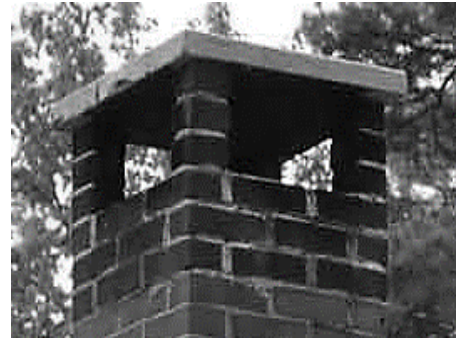
Concrete Cap Chimney Top
