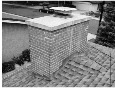
Clay Liner Cover
